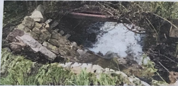
Bridge on the Corkscrew
