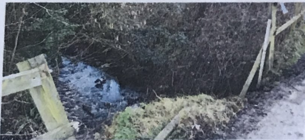
Bridge on Ridgeway lane.
